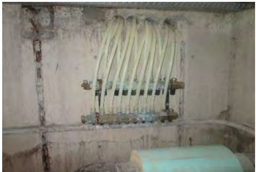
Figure 12 - Snowmelt; confined space - improved safety and control
