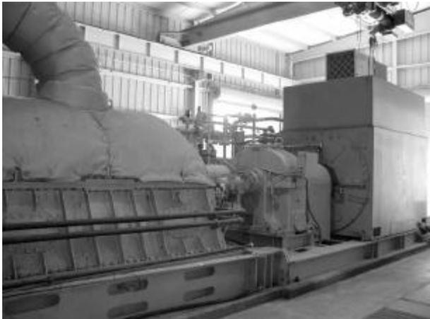
**Figure 10.** *The condensing turbine.*
