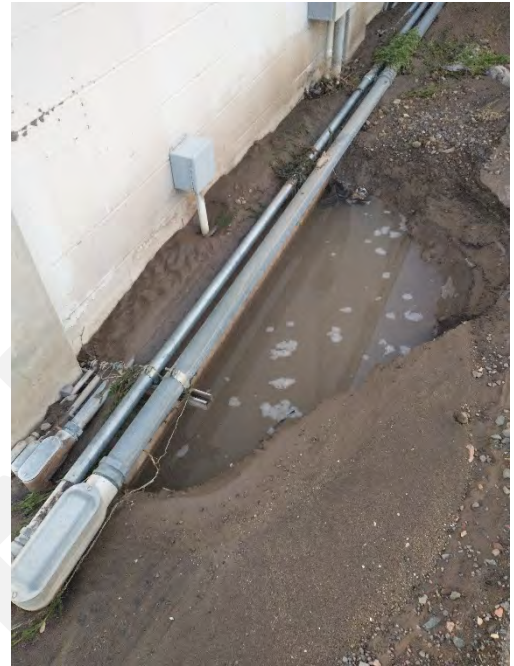
Figure 1 - Main pipe from Well #6 ruptured at building foundation footing, from incident on September 7, 2022
