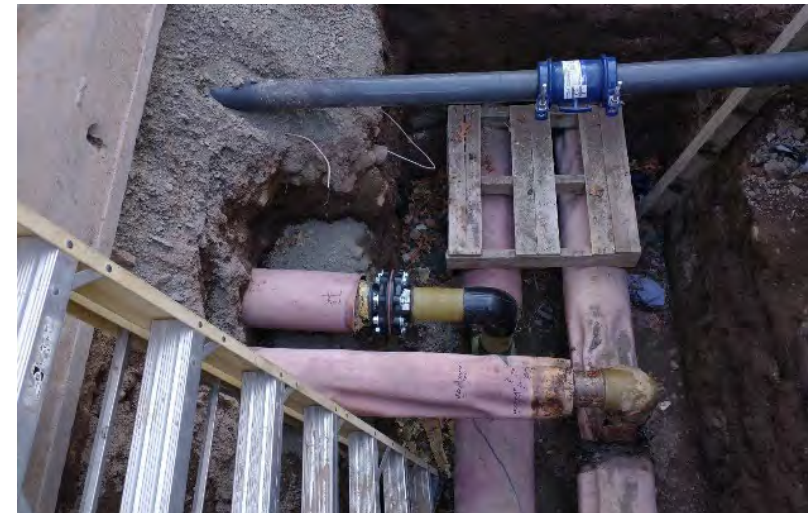
June 2021- Valve and pipe failure causing temporary residence hall closure.
