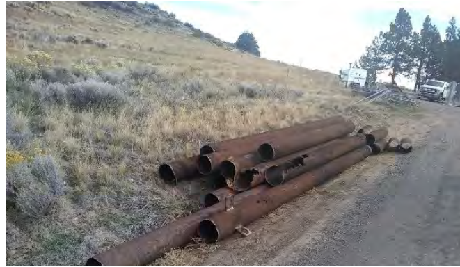
Winter-Spring 2022- Well #5 shut-down due to corrosion and failing pipes putting campus at risk of closure.
