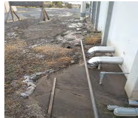
Sept. 2022- Main pipe from Well #6 ruptured at building foundation, causing closure.
