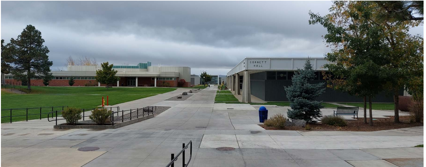
Excessive paving outside of Cornett Hall
