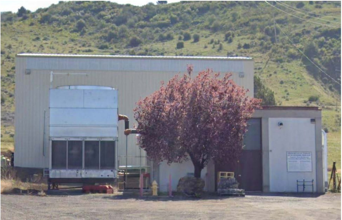
Large Geothermal Power Plant
