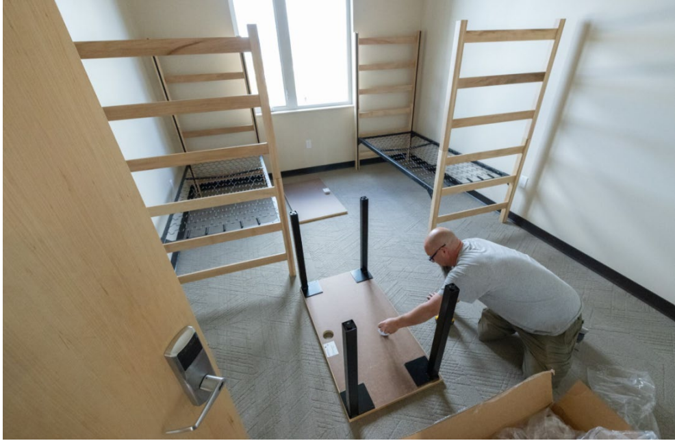
Photo: Installation of furniture into New Student Housing. (Photo Credit—Chris Santucci)
