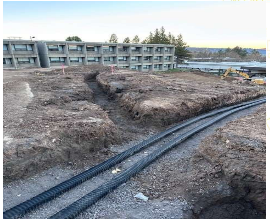
Snowmelt Main Supply In Trench South Hillside
