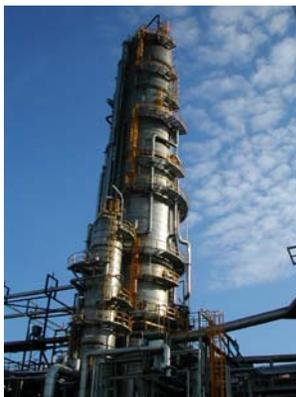
These different molecules are partially purified by **fractional distillation** where lower boiling liquids are preferentially boiled off and separated from higher boiling substances. This process does not separate out pure compounds, but it does separate the crude oil into separate fractions with similar boiling points.
